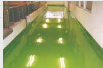
食品、医薬プラント等の塗り床 Anti-corrosion flooring for foodstuffs and pharmaceutical plants, etc. (coating)
